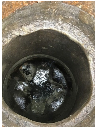
MH After Repair
