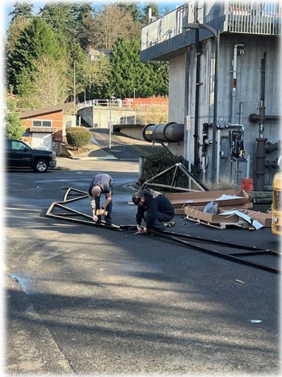
Start of project carport.
