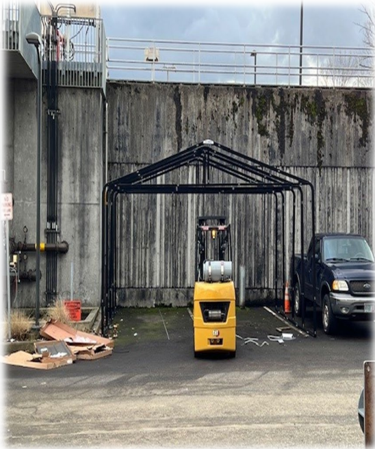
Carport is up.
