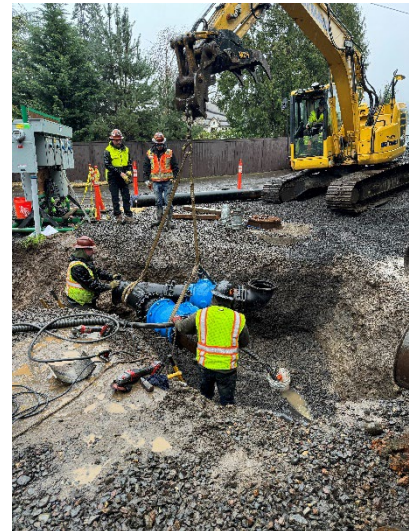
Lift Station #2 Valve Install
