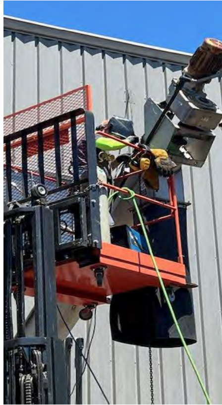
Maintenance welding the auger back in place.
