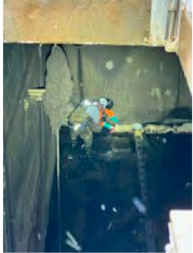
Digester 2 aeration line repair
