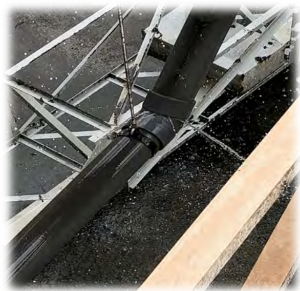
3) Clarifier #1 scum pipe leak
