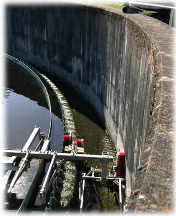
5) New clarifier brushes (with supervisor)
