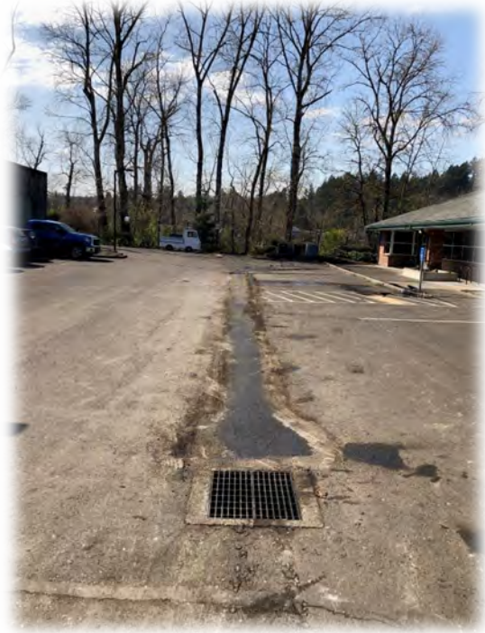
6) Plant parking paving
