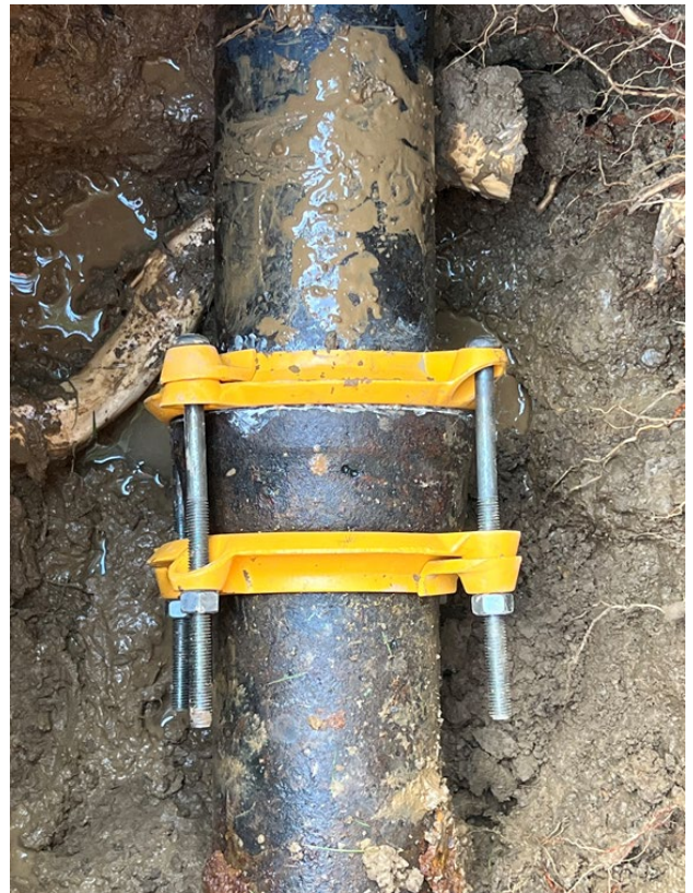
Photo 7: Bell-joint repair on Glen Echo
