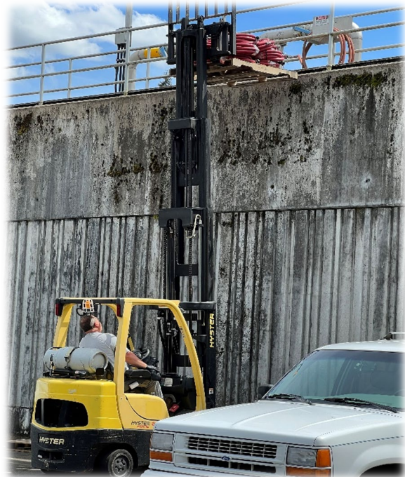
Fresh batch of hoses being placed on Aeration basins.
