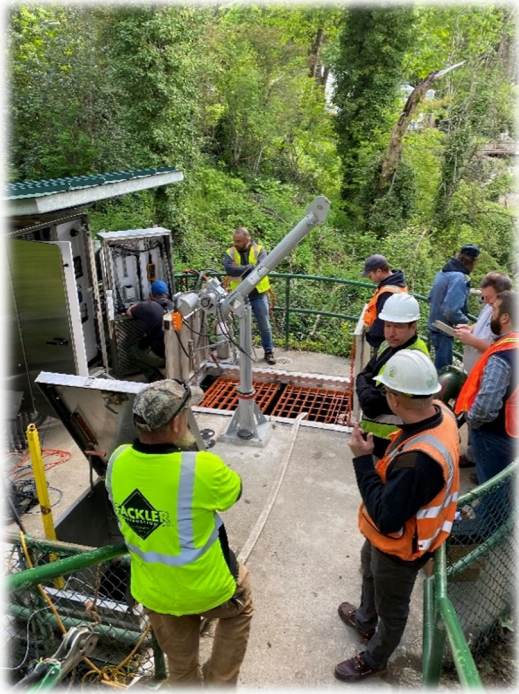
Lift Station 5 shakedown on May 11 th
