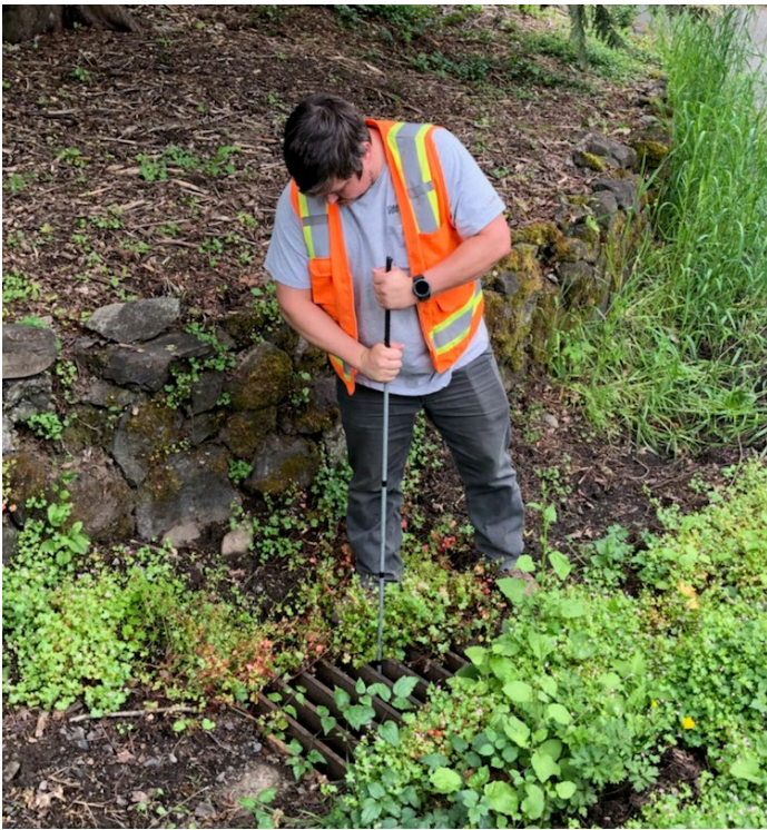
Photo 1: Zone 5 stormwater system work
