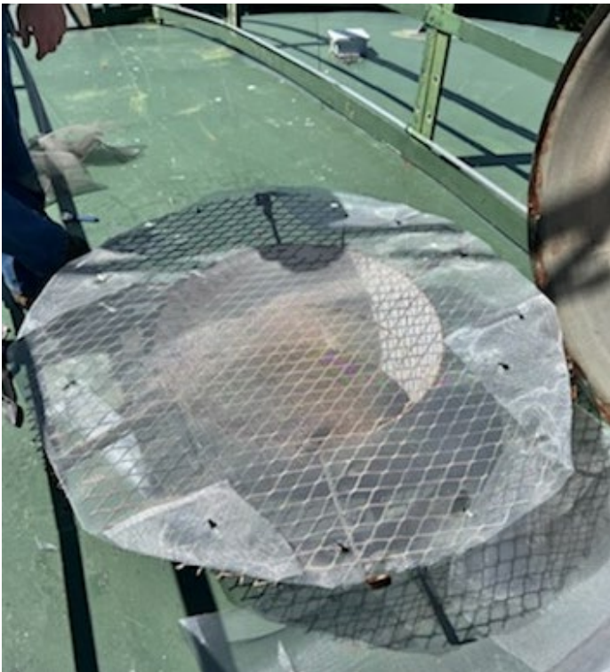
Photo 3: Finer vent screen installed
