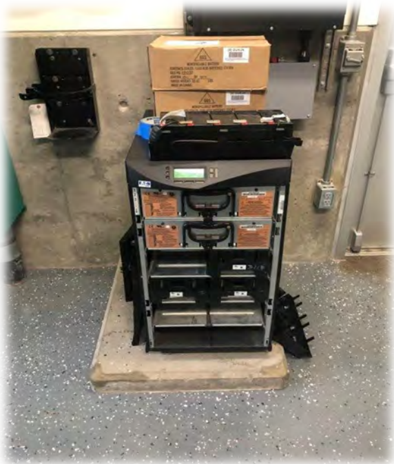
(7) UPS Battery Replacement
