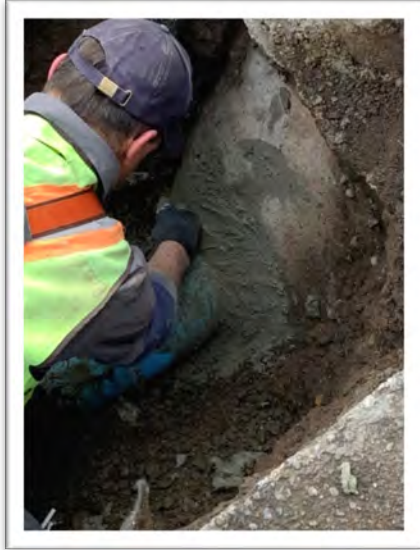
1. Pipe being grouted in.
