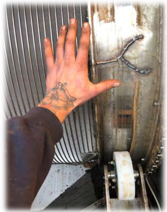
4) Drum Screen Weld (Jayson's hand)
