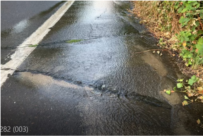
Photo 7: Service line leaking on Roethe Road
