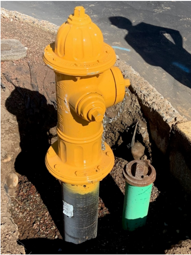
Photo 5: New fire hydrant on Fircrest Court
