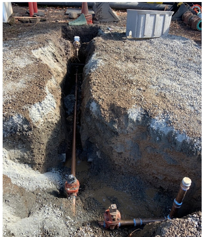
Photo 4: New 1.5-inch water service and flush-out
