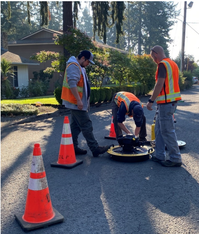
Photo 1: Setting up smoke testing machine
