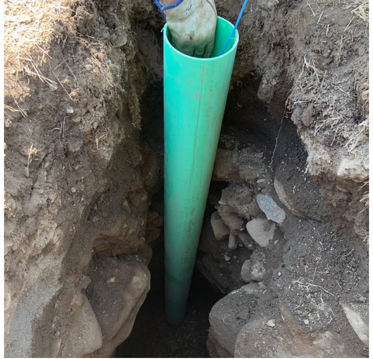
Photo 6: Tracer wire installed on 24-inch main
