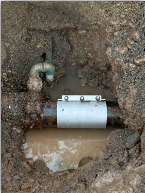
Water main after repair band was installed.
