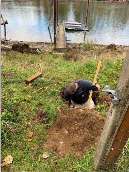
Sewer manhole found 2-1/2' deep (10/21/20)
