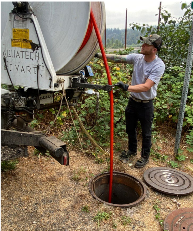
Photo 1: Line segment cleaning in basin 2B
