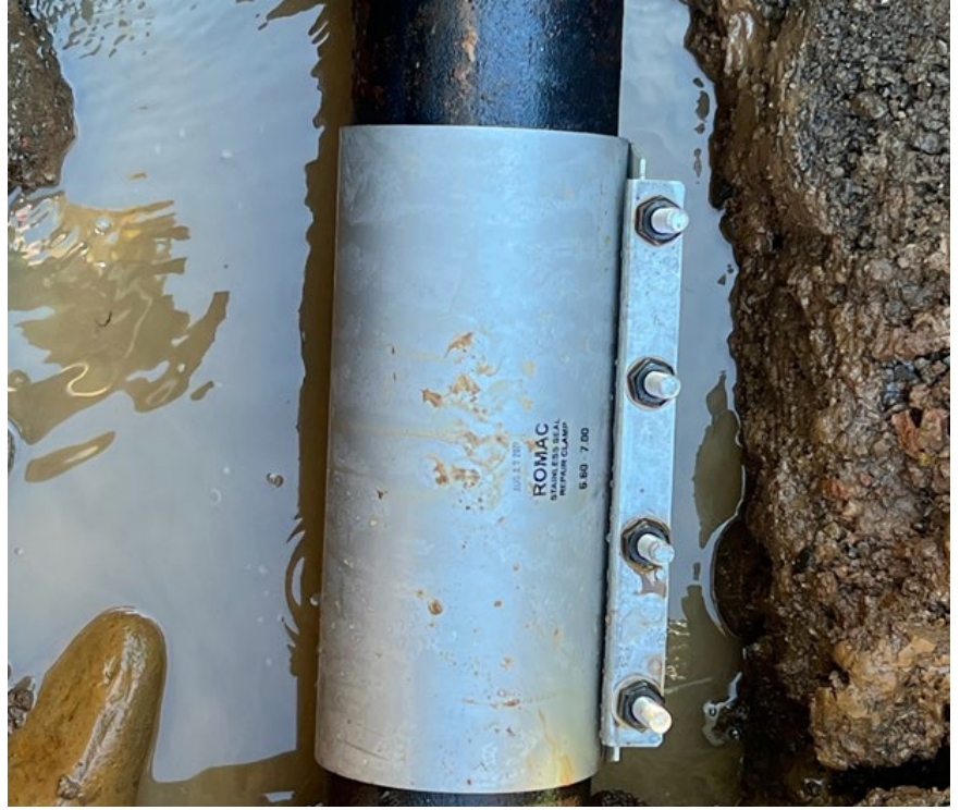
Photo 7: Leak repaired with full-circle clamp
