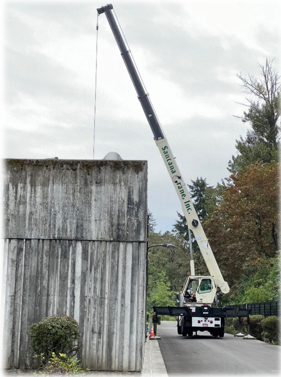
Crane Removing Aeration Basin Mixer
