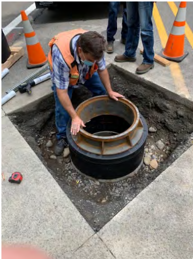
(8) manhole placed on top and for final leveling.
