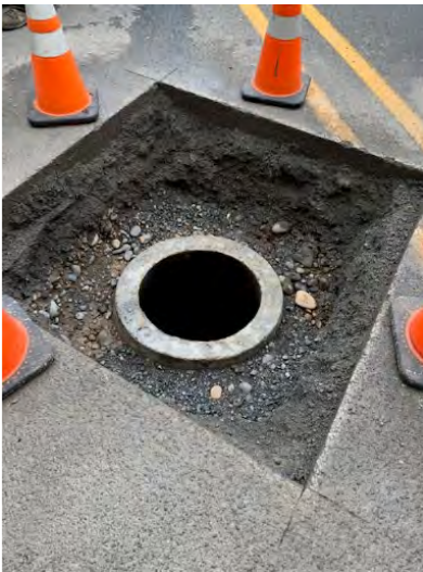
(5) top is removed and cleaning preparations are made.
