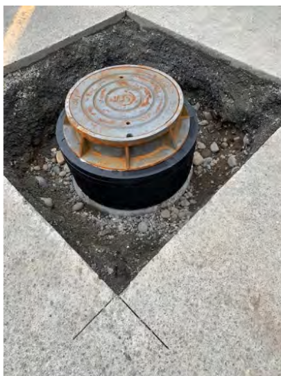
(9) all that is left to do is back fill and pave.
