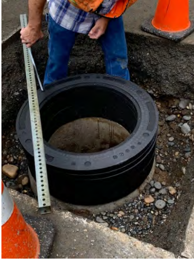
(7) more pieces are glued and leveled with road.
