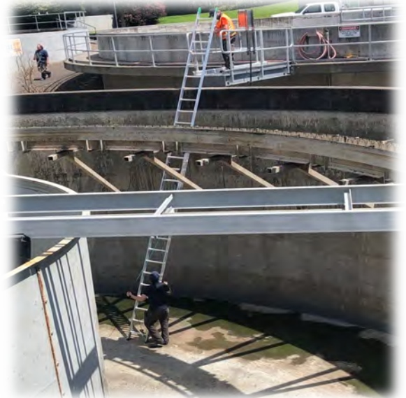
4) Clarifier #1 for pipe repair
