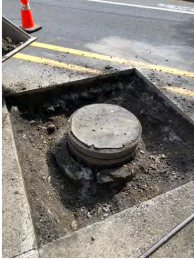
(4) Crews dig out around manhole.
