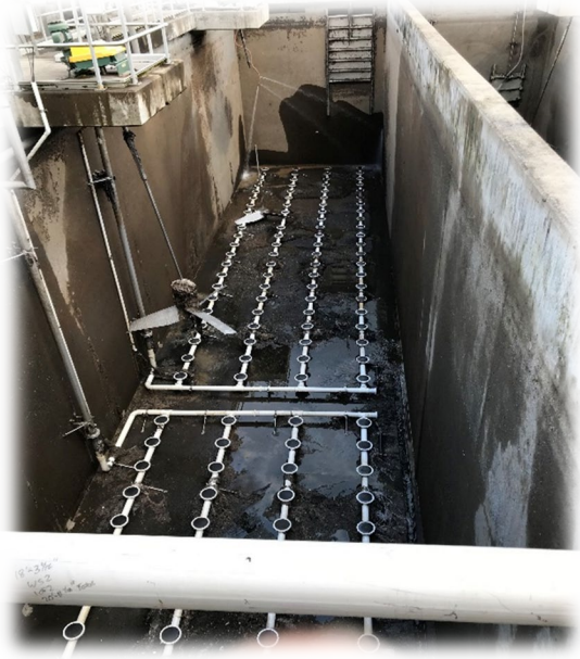
1) Aeration Basin #1 drained
