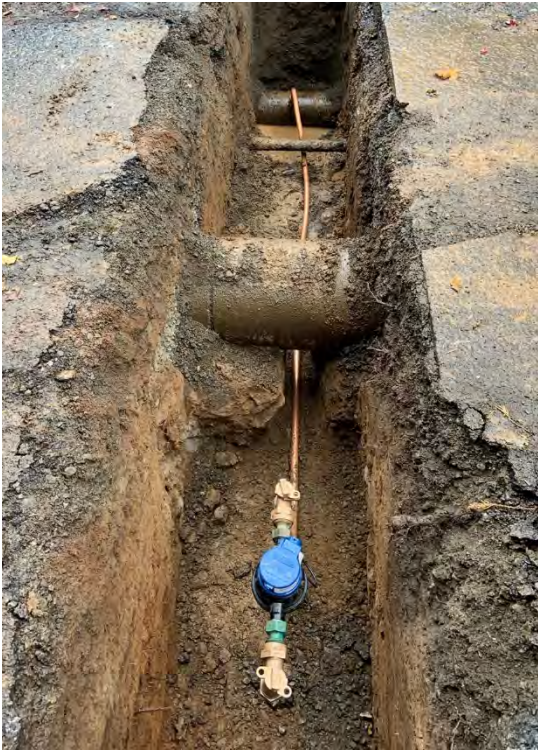
Photo 5: New water service on Risley Ave.
