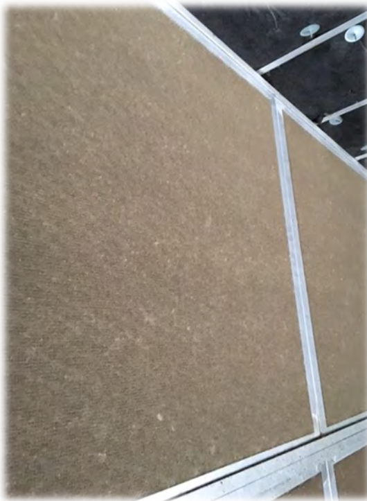
3. Headworks air handling screen before.
