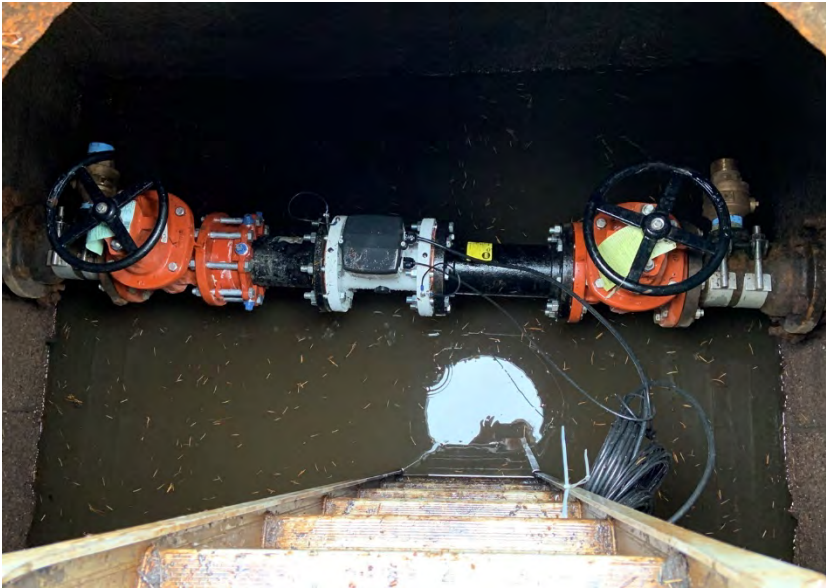
Photo 7: Newly installed 4-inch water meter
