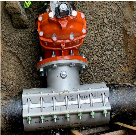
Photo 8: Tie-in for new subdivision
