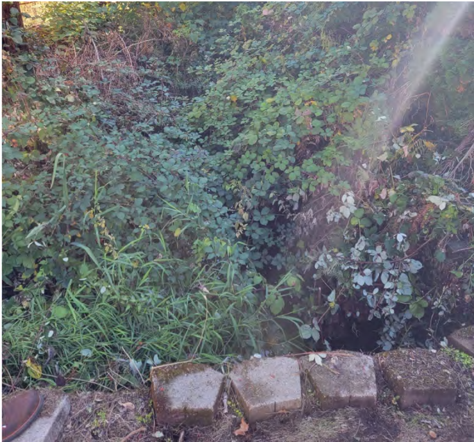
Photo 1: Drainage ditch at Laurie and Anspach pre-work
