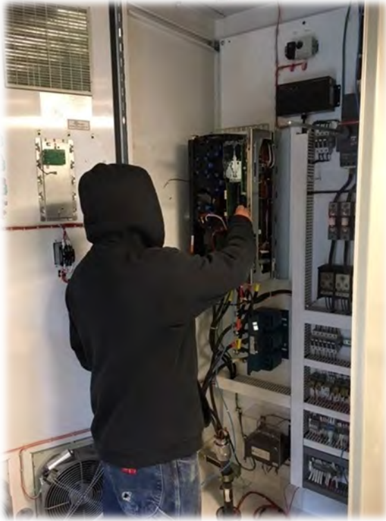
5. Tice electrician working on Influent VFD's
