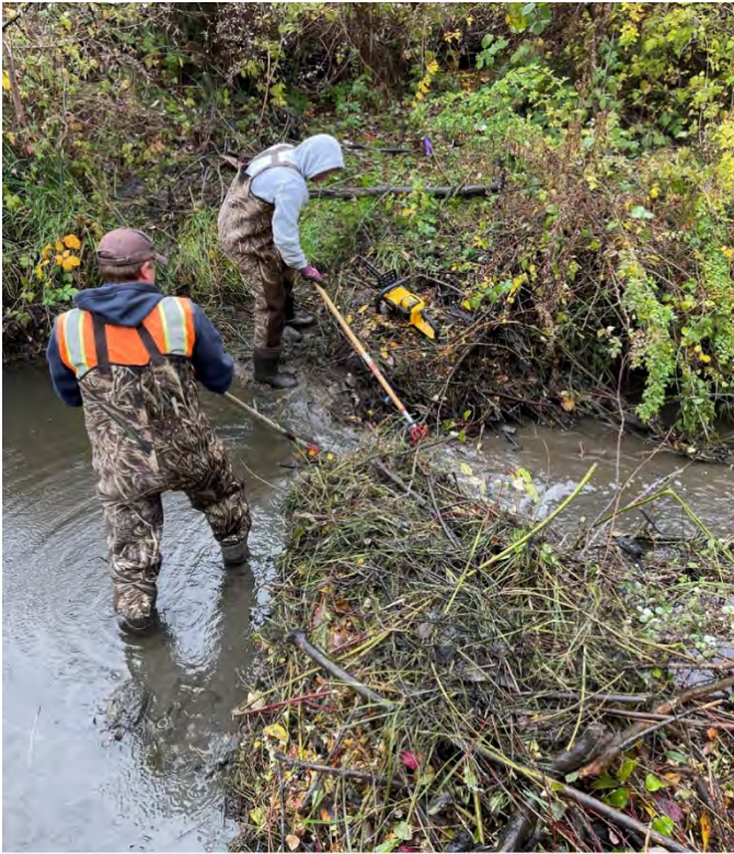
Photo 3: Removal of nutria dam at Stringfield Park
