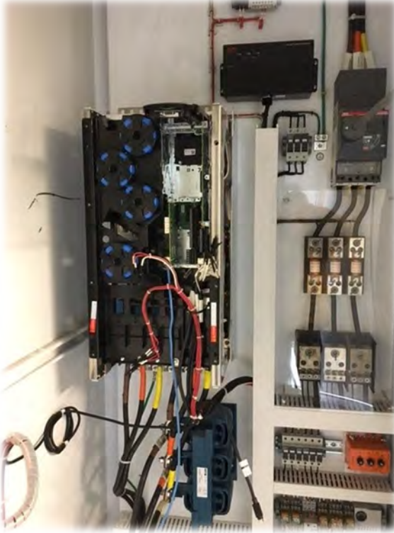
6. Finished product of VFD upgrade.
