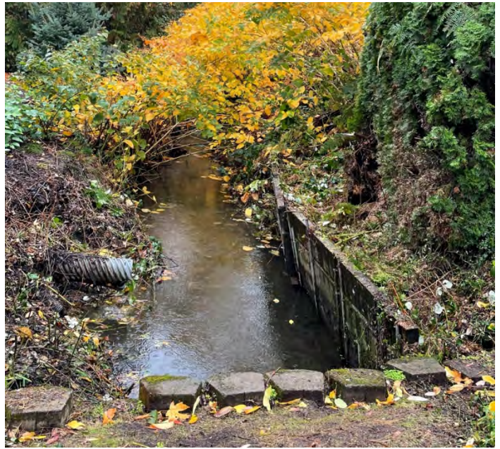
Photo 2: After ditch clearing
