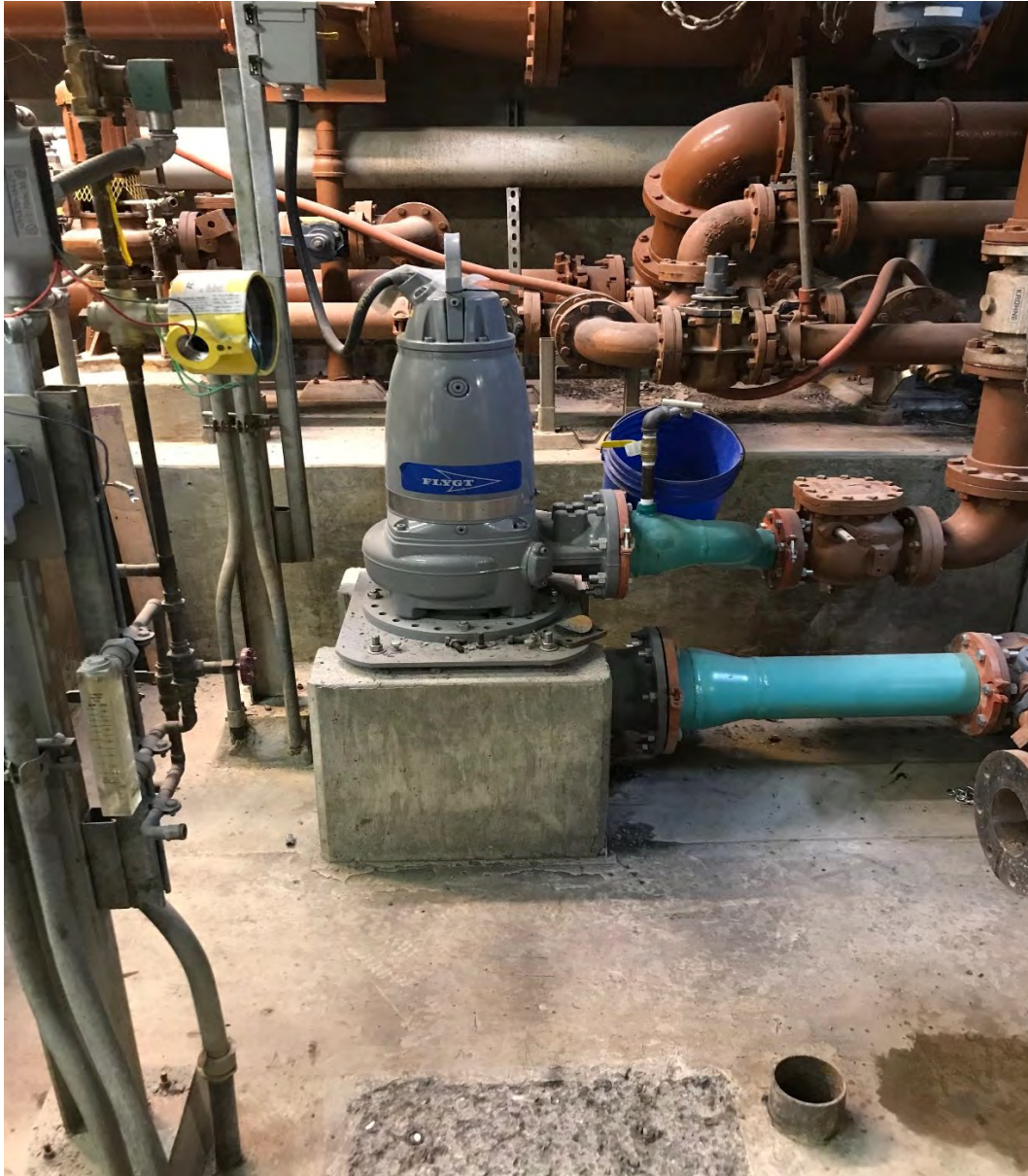
Photo 1 The newly installed and operating Return Sludge Pump.
