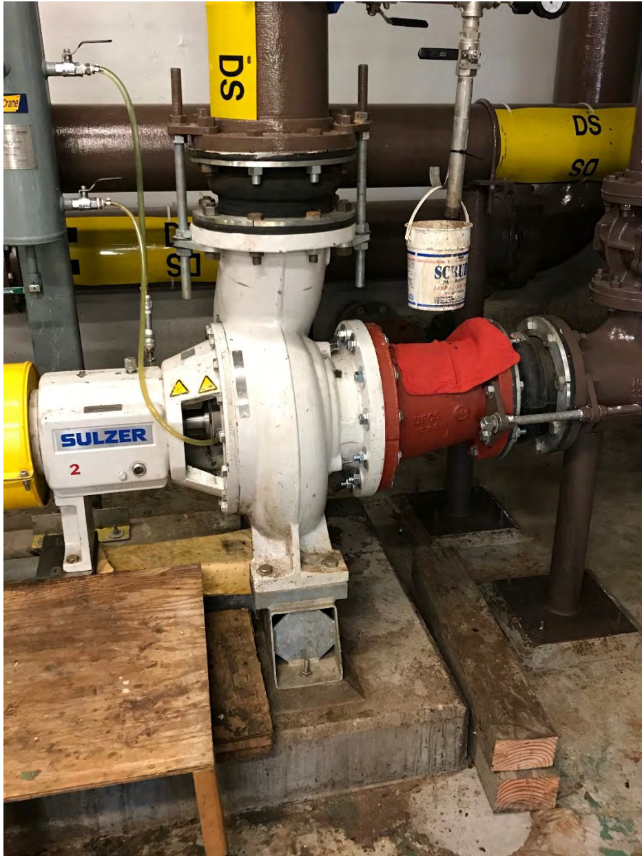
Photo 3 The new cone installed on Digester Mixer Pump #2
