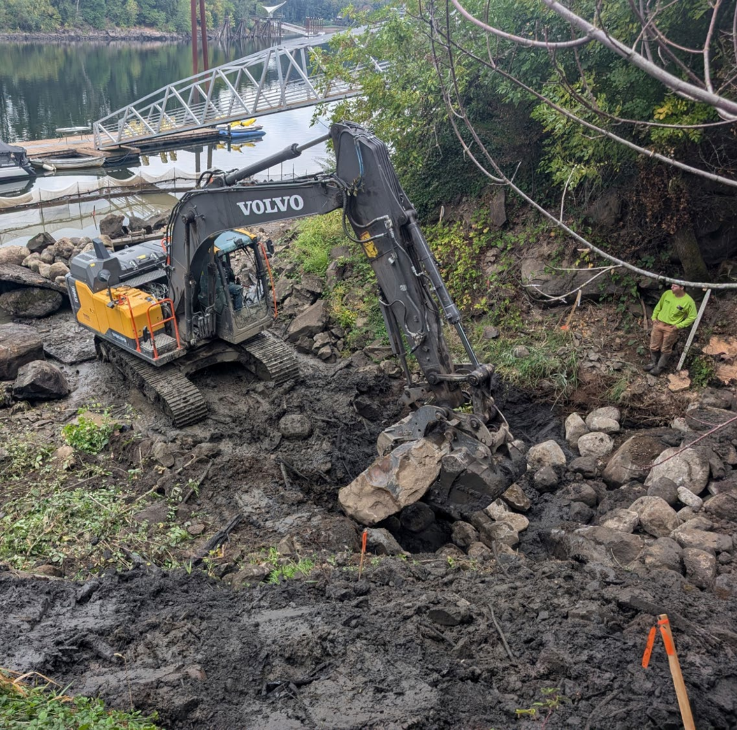
Engineered streambed material and roughened channel.
