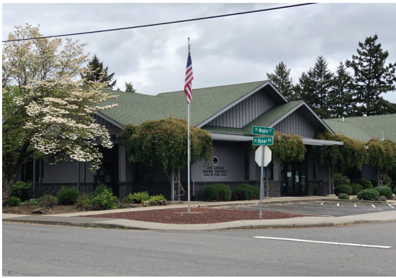
Administration Office 14496 SE River Road Oak Grove, OR 97267
