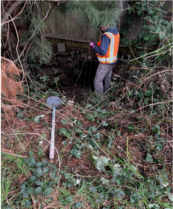
Photo 2: Catch basin located down in a recess
