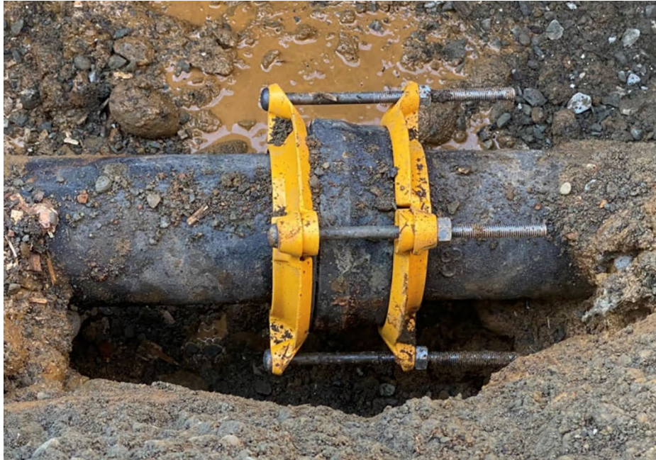
Photo 9: Bell-joint repaired!
