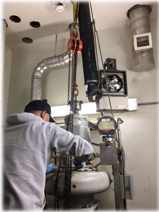
Maintenance pulls pump at Lift Station #3.
