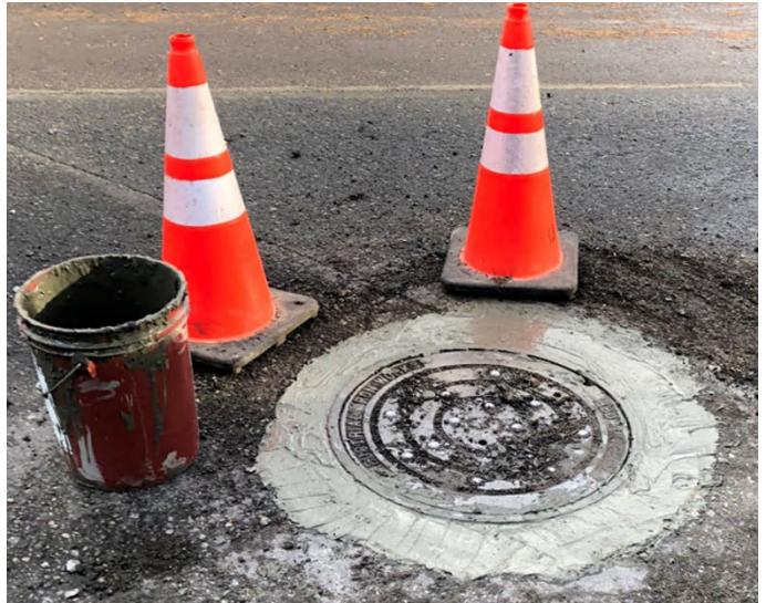
Photo 6: Spot repair of manhole
