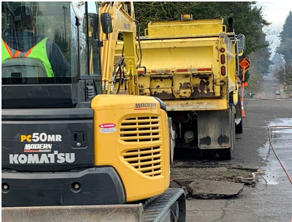
Photo 10: Temporary road repair at Hull and Rose
