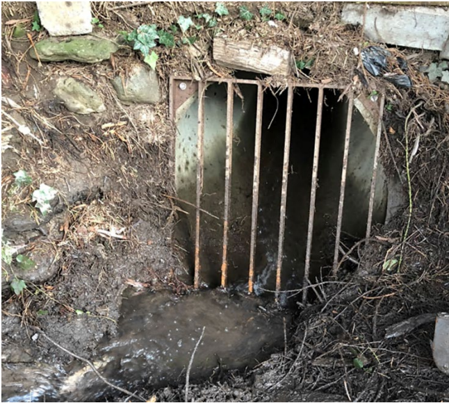
Photo 3: Cleaned catch basin
