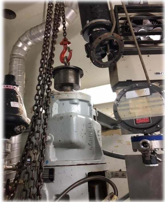
Pump ready to be pulled out.
