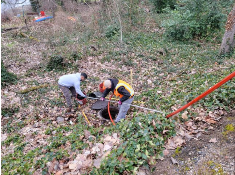
Photo 4: Collection system cleaning along an easement
