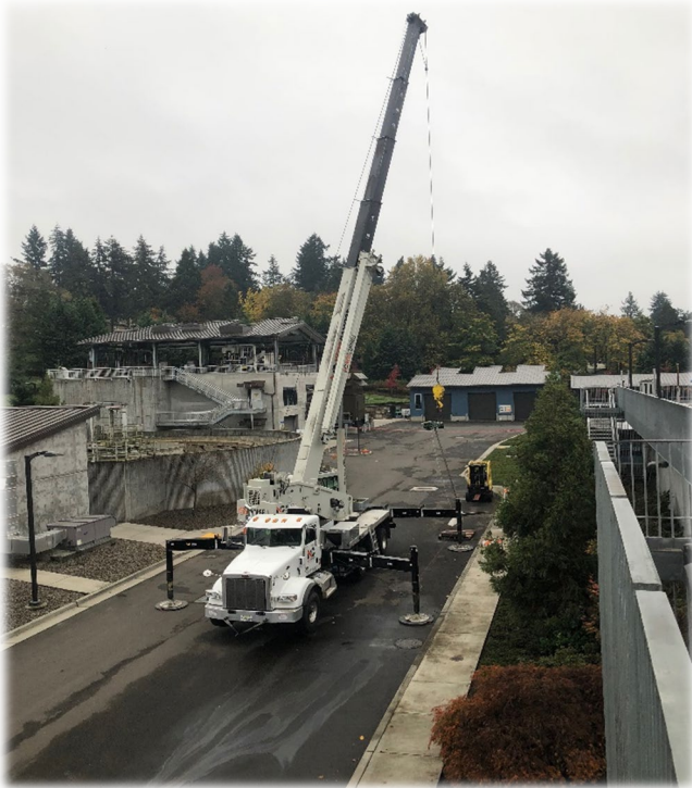
Lifting the Aeration Basin mixer.
