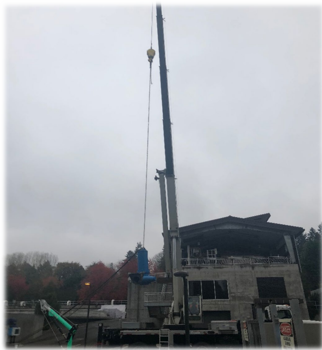
Installing the Influent Pump
