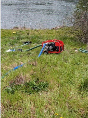
Trash Pump Bybass
