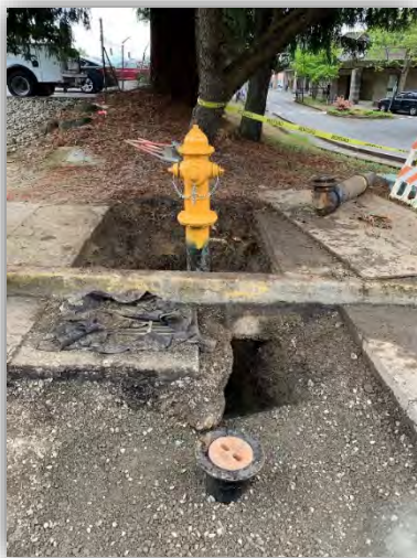
Hydrant after installation.
