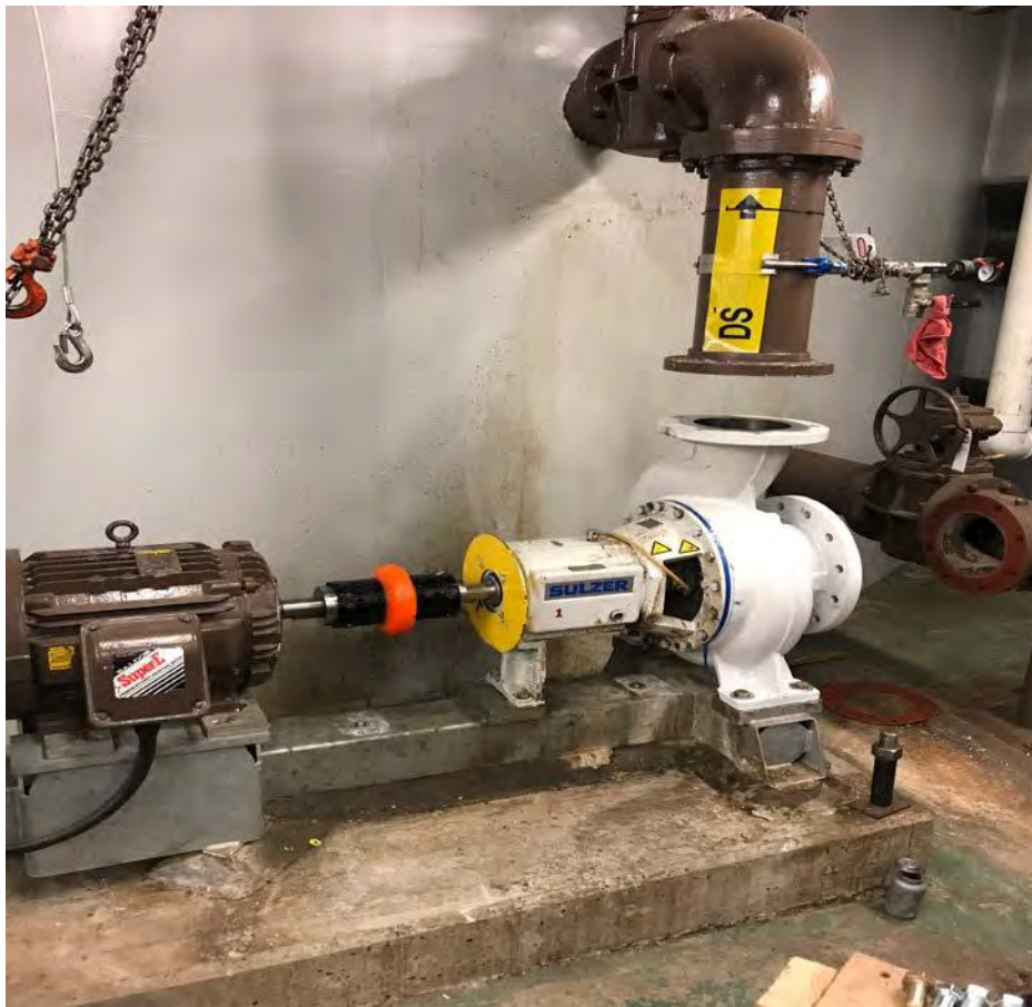
Digester Pump #1 repair in progress with volute installed
