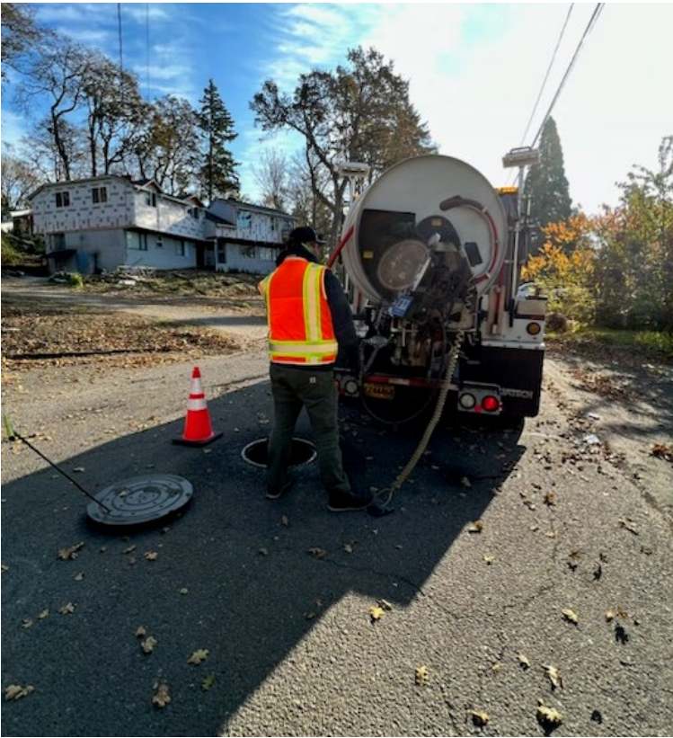
Photo 1: Routine hydro-cleaning work in Basin 2C
