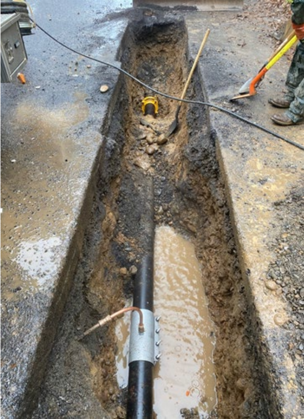
Photo 3: Watermain leaks repaired on Oatfield
