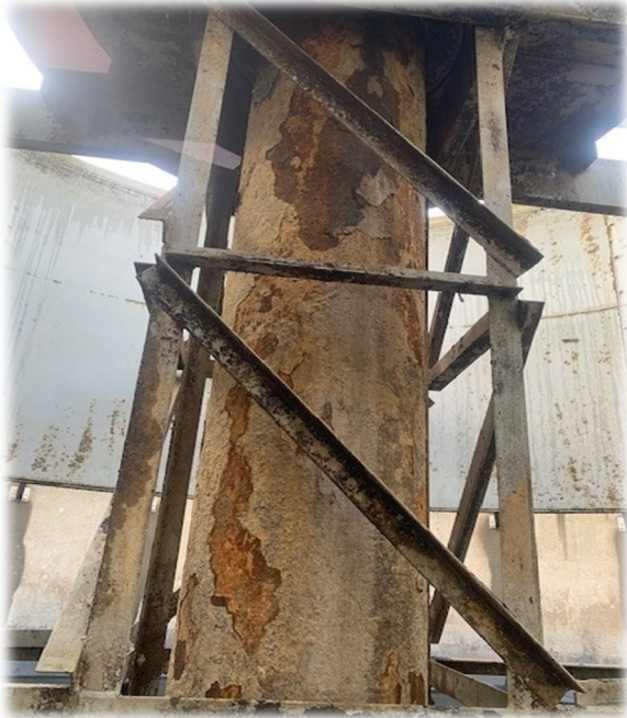
Center Pipe Structure of Clarifier #1
