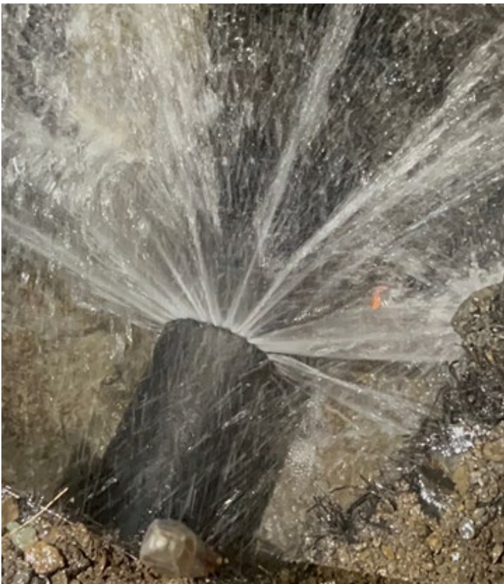
Photo 5: Radial split on 6-inch cast iron
