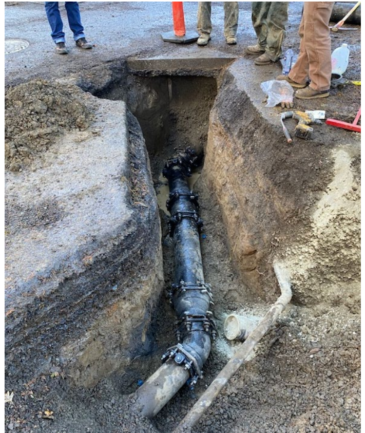
Photo 6: Watermain tie-in for Aldercrest project
