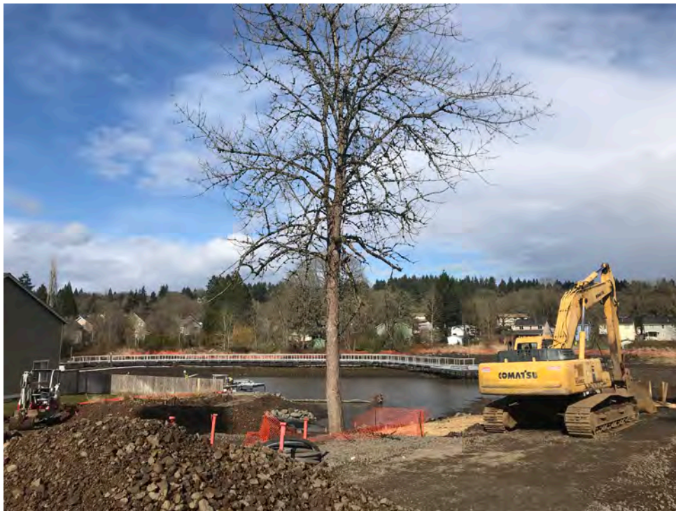
Oregon Ash During Construction
