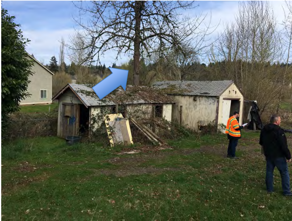
Oregon Ash Pre-Construction
