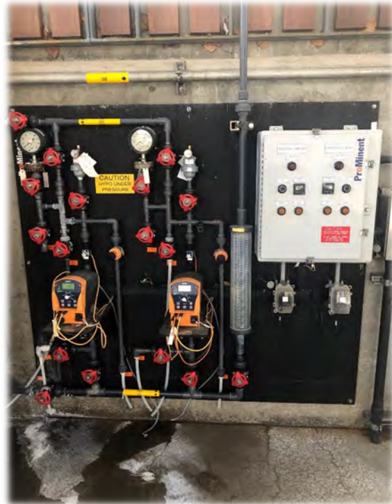
Hypochlorite dosing pumps.
