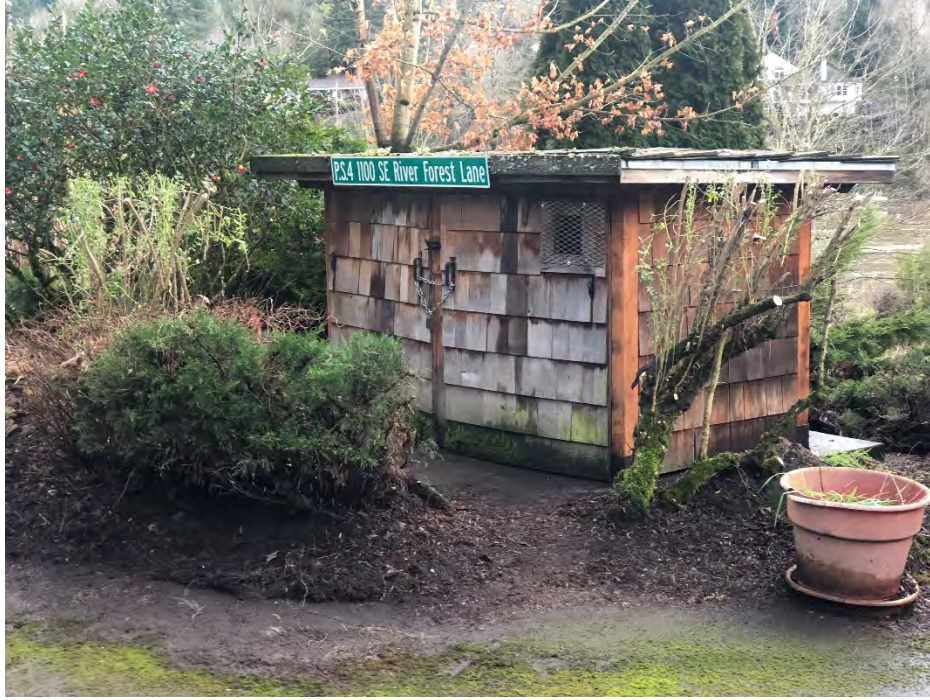
Pump Station #4 Landscape Clean Up
