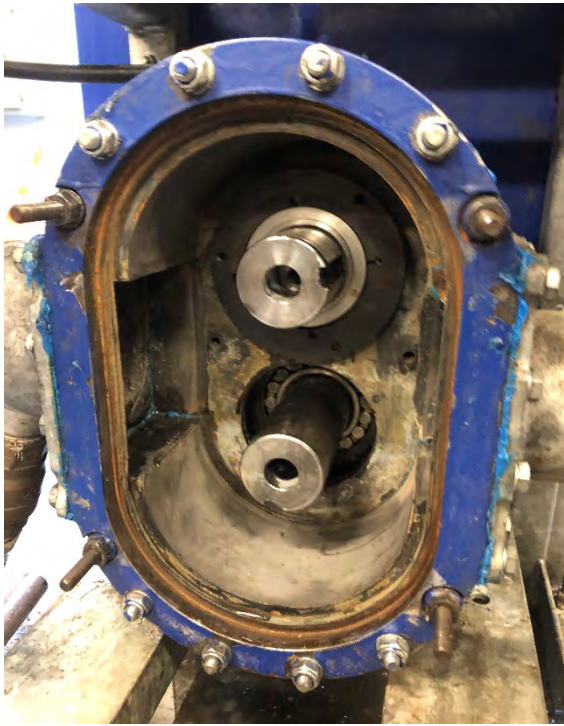
Digested Sludge Pump Seal Replacement
