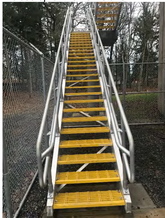
A close up of the new stairs.
