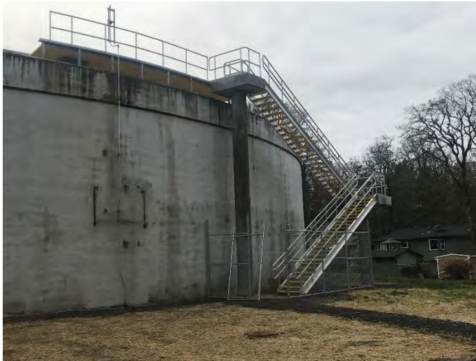
This shows the new stairs and landing at the top
