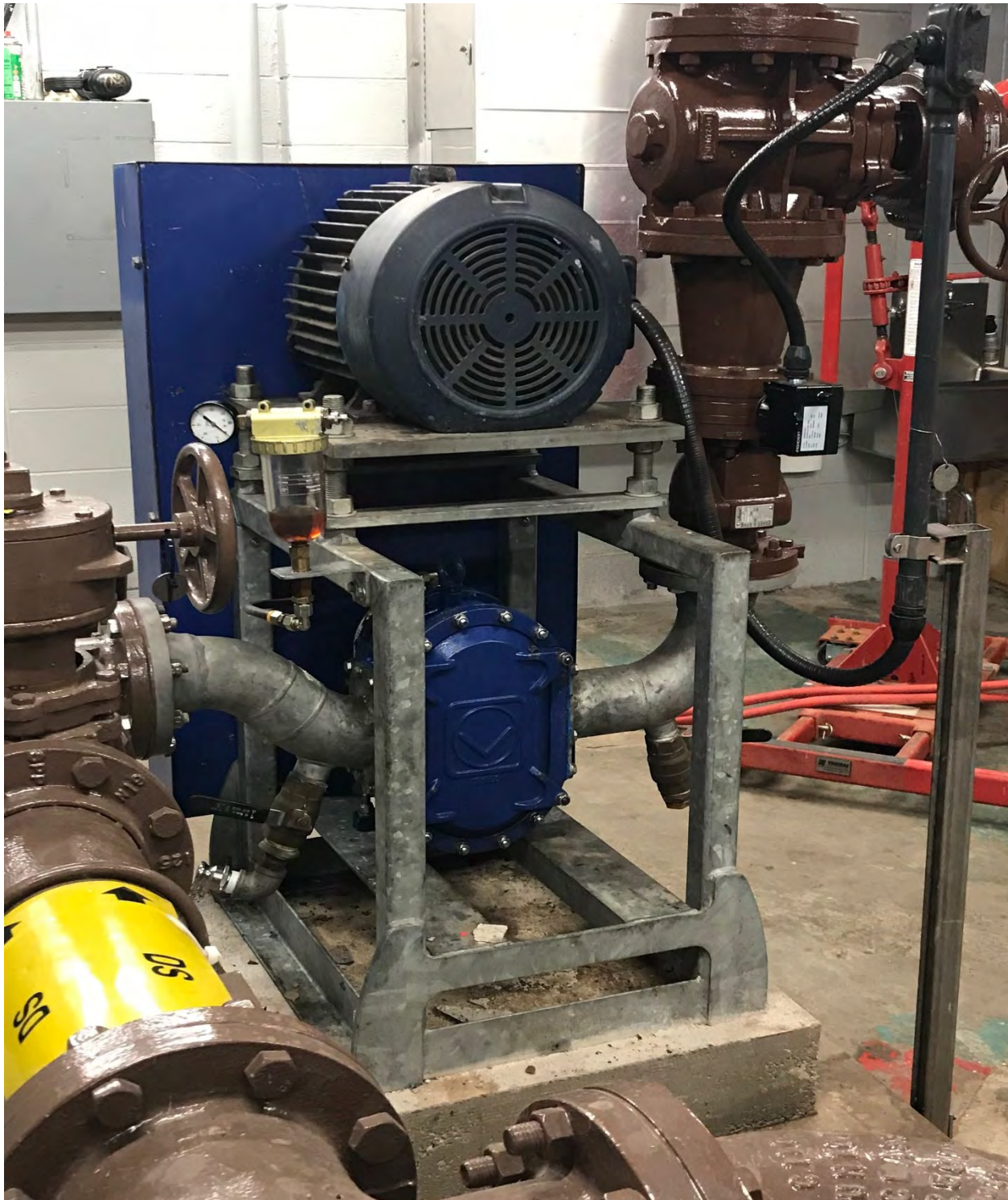
Photo 2 Rebuilt Vogelsang Digested Sludge Feed Pump
