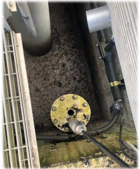
Level Detector calibration
