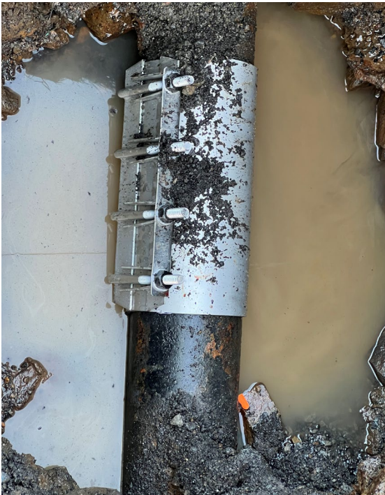
Repaired main at Oatfield north of Park Avenue
