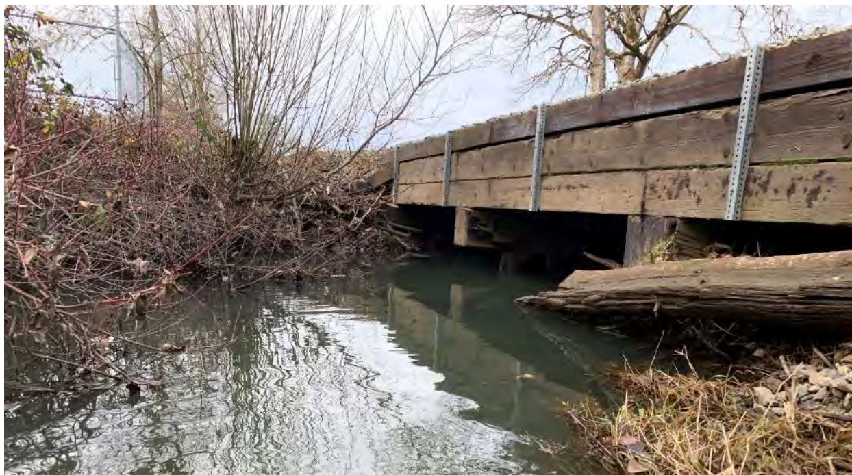
Figure 43. Downstream railroad bridge crossing MSC at the start of Reach 5 (rKm 3.82).
