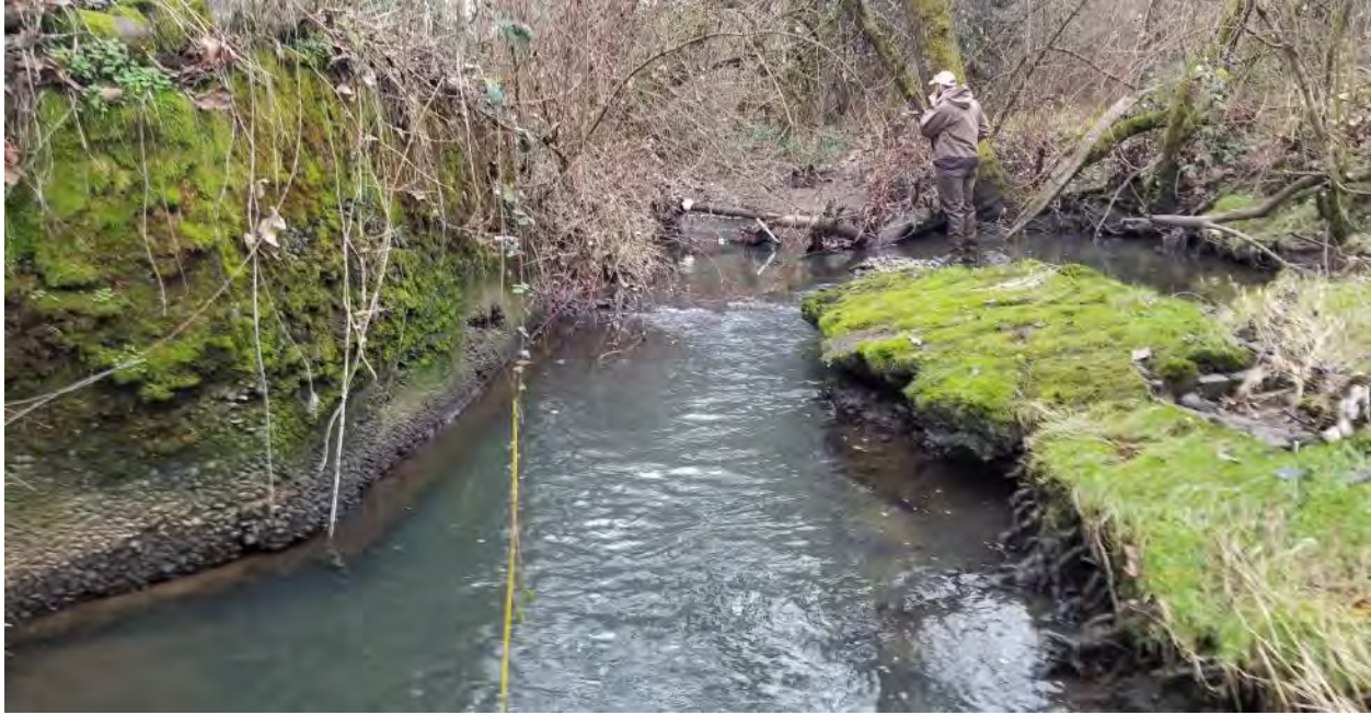
Figure 32. Historic bridge abutment in channel constricting flow near rKm 3.6.
