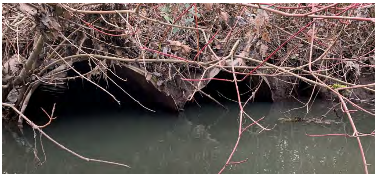
Figure 44. Culverts connecting Dean Creek to MSC near rKm 3.82.
