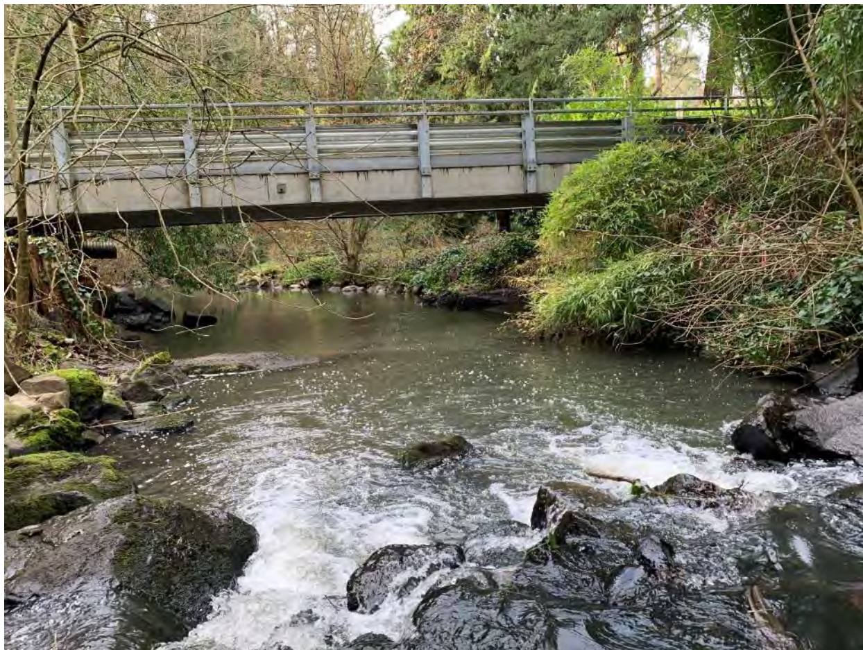
Figure 18. Keuhn Road bridge crosses the channel near approximately rKm 3.55.
