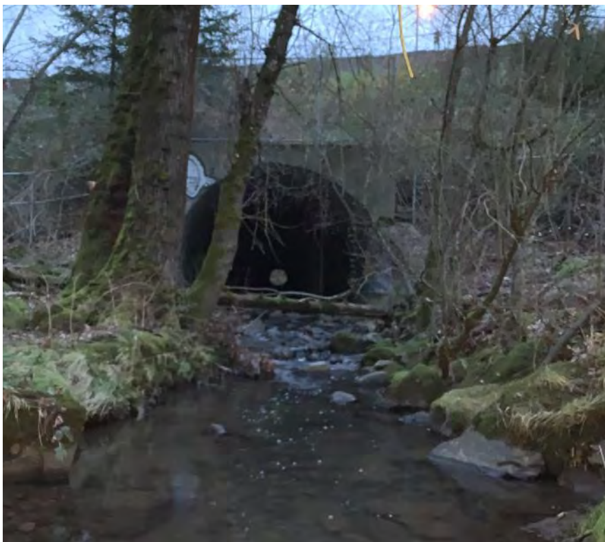
Figure 48. I-205 culvert outlet; the upstream extent of MSC Reach 5.
