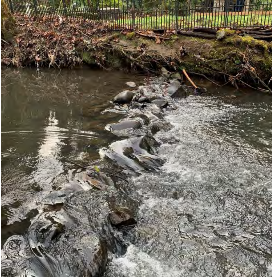
Figure 21. Example of small, man-made rock weirs within the Kellogg Creek channel in Reach 1. There are numerous of these present throughout the study area (and likely downstream of surveyed portion of reach as well).
