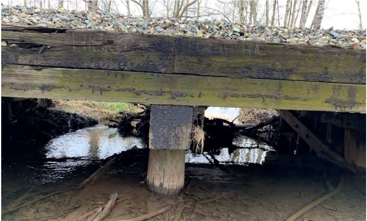
Figure 45. Upstream railroad bridge crossing MSC at the rKm 4.09.
