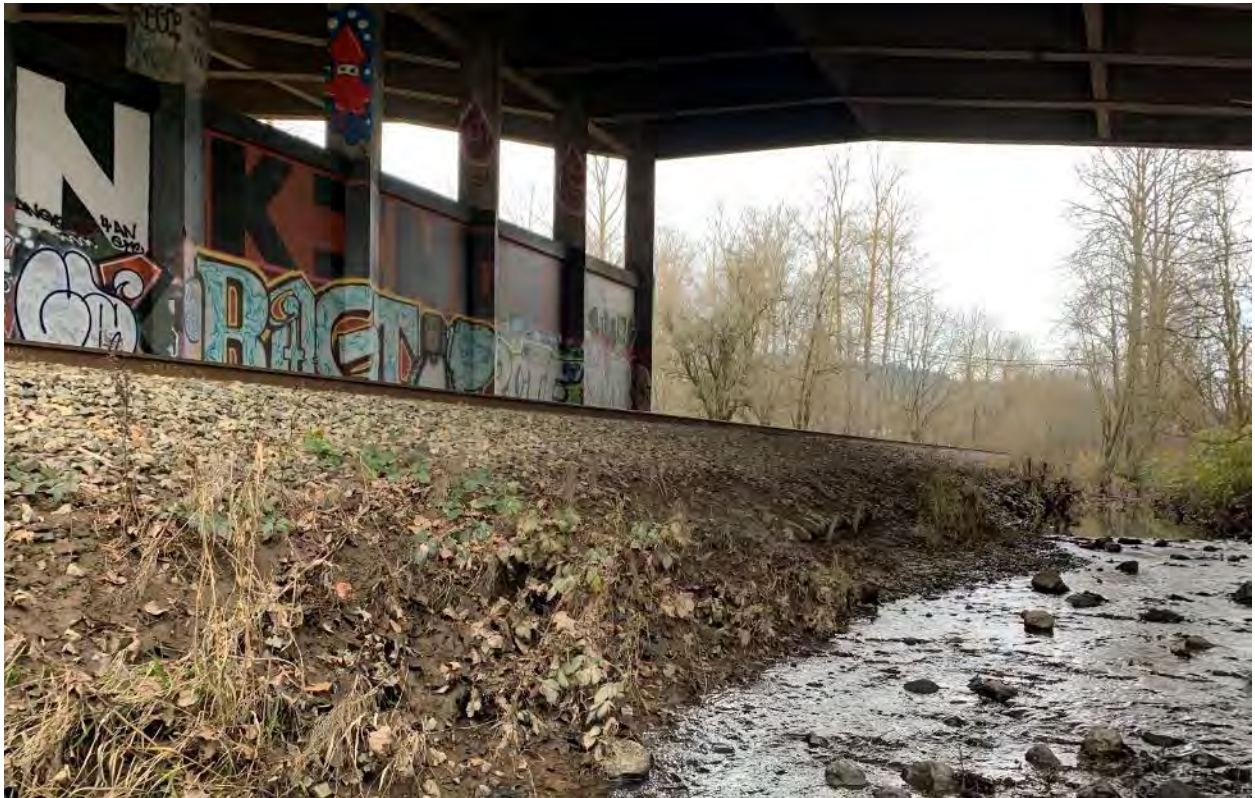
Figure 46. MSC adjacent to railroad, under the large 82 nd Ave/Hwy 213 bridge.
