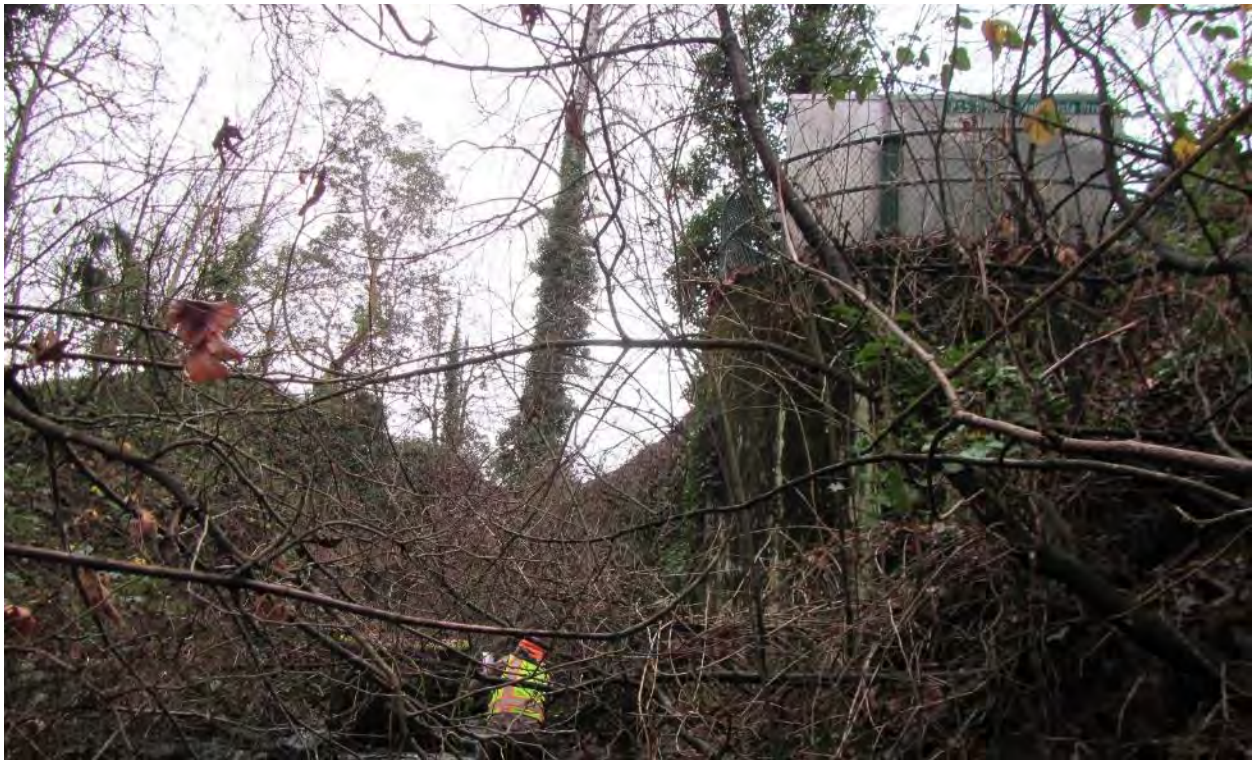
Figure 61. Standing in Boardman Creek and looking downstream at the large stormwater/sewerline infrastructure located on the river right bank near approximately rKm 0.1.
