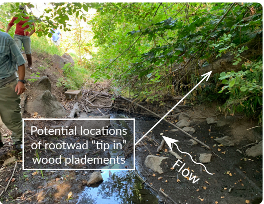
Rootwad “tip in” wood placements, emulating natural large wood recruitment to a channel, are proposed along the north bank and could incorporate existing trees where feasible.
