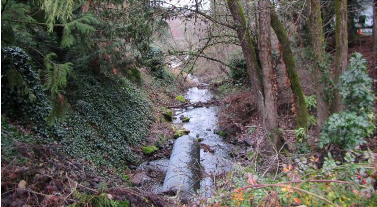
Figure 78. Standing on SE River Forest Drive, looking downstream at River Forest Creek channel out to confluence with Willamette River.
