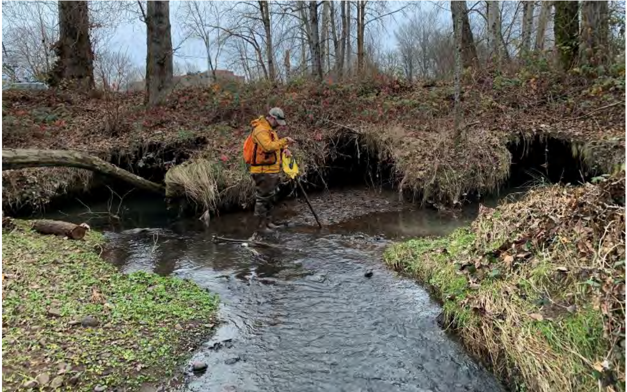
Figure 47. Series of 3 culverts under 84 th Ave near rKm 4.58 in MSC Reach 5.
