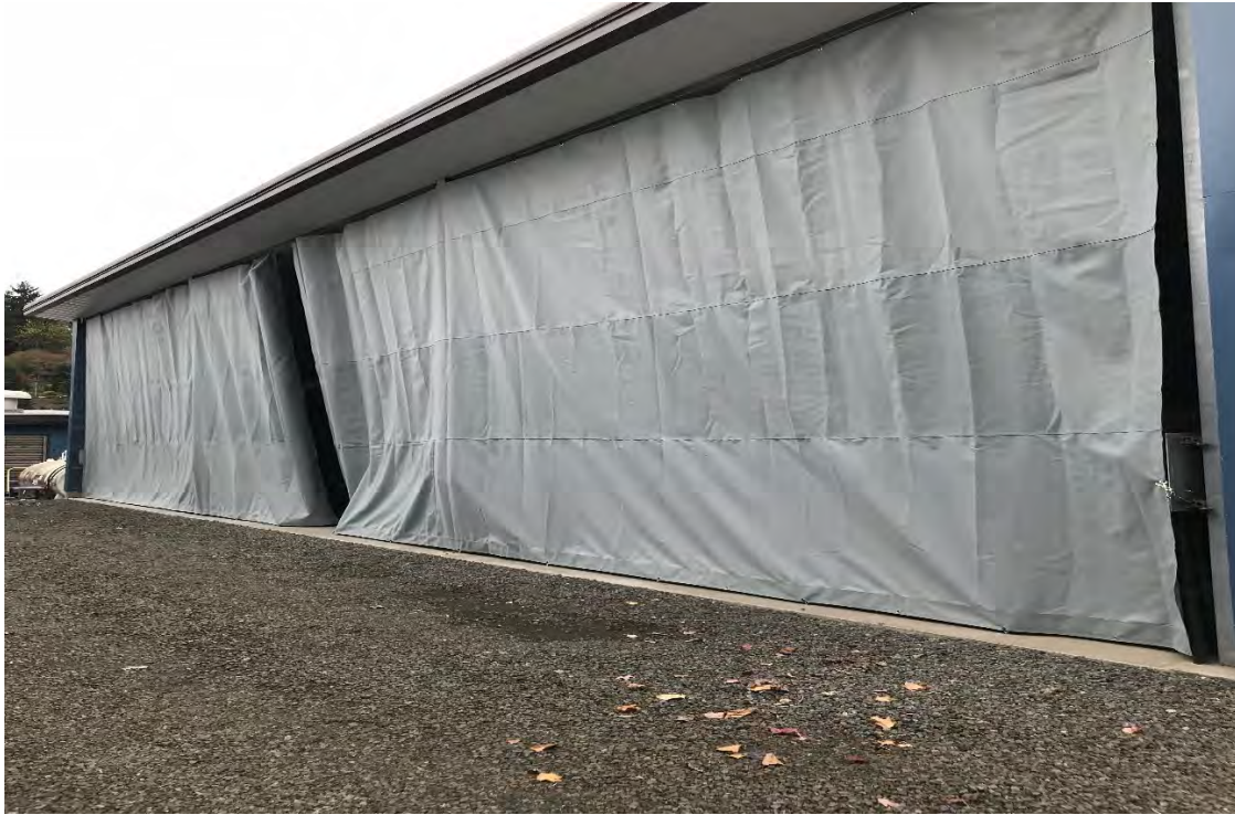
Photo 3 New Tarps for Aeration Blowers.
