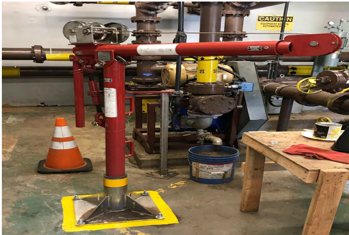
Photo 2 The new lifting davit in digester room
