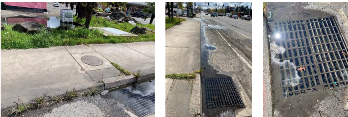
Photos of ODOT-maintained catch basin along McLoughlin Blvd.
