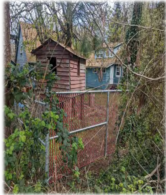
Fence after repair.
