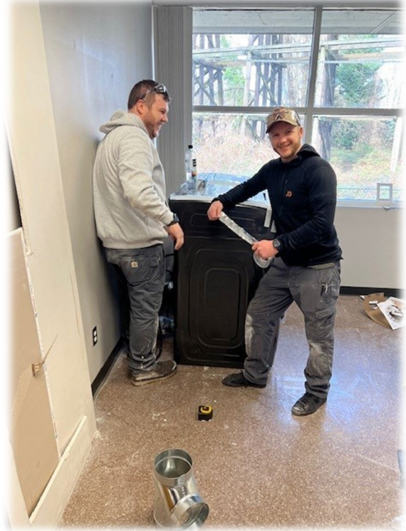
Matt and Abe Installing the Dryer Vent.
