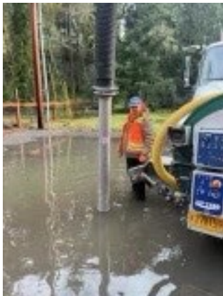
SSO Cleanup in progress
